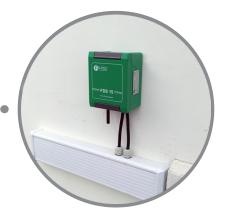
For monitoring the fine dust content at factory premises of the company SNF Floerger a FDS 15 has been mounted at the outer wall of an office building. By means of this outside installation the own production shall be controlled as well as the actual fine dust content of the ambience shall be monitored.
